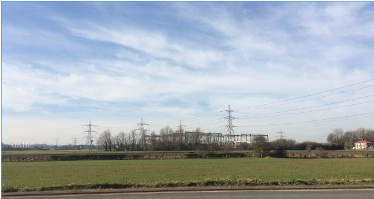
Plate 25: Views towards Creyke Beck NGET Substation from Dunswell Road.
