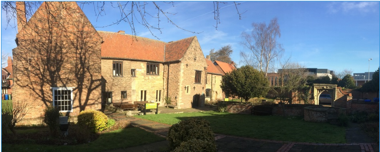
Plate 10: Converted building at the Friary Scheduled Monument site
